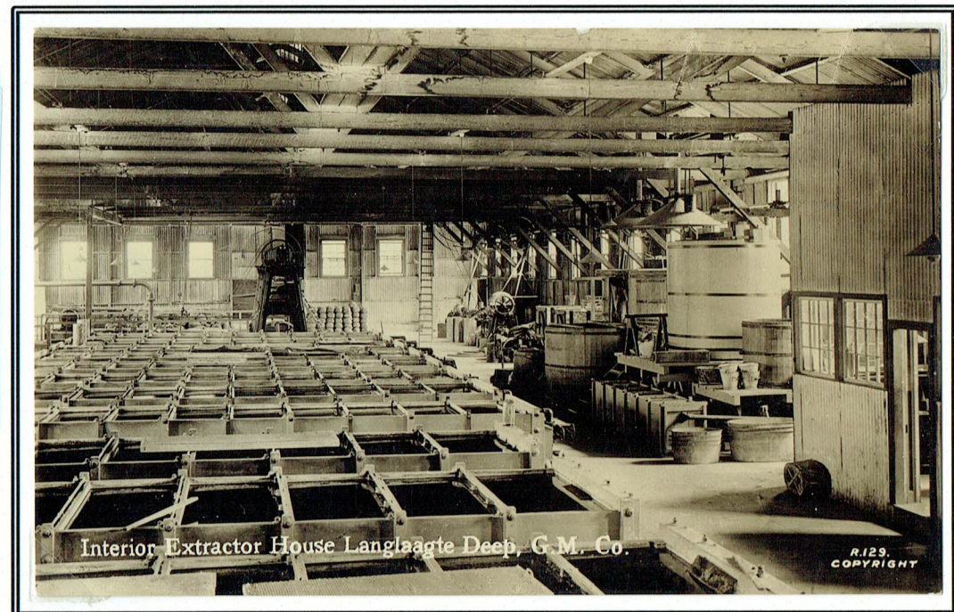
Interior of the Extractor House
