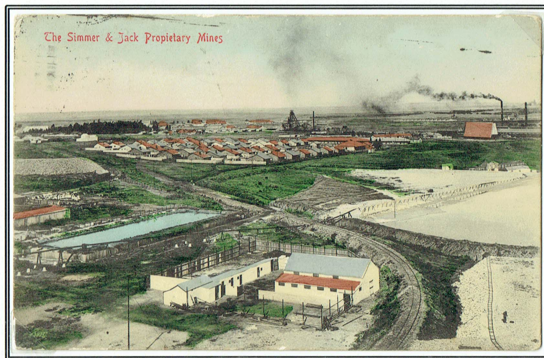
Overview and surface workings of the Simmer and Jack gold mine Published by Sallo Epstein & Co, Durban, DB in green with number serial number 2108
