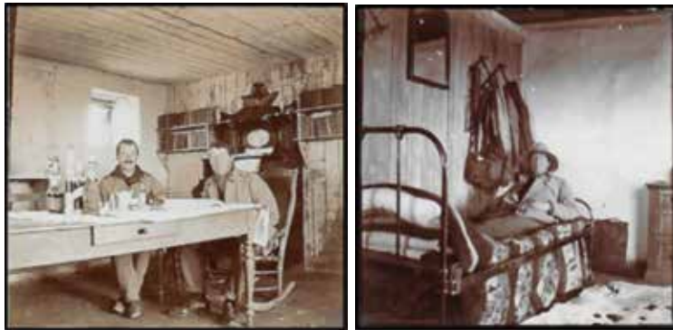
Fig.14. Inside the Harrismith Blockhouse
