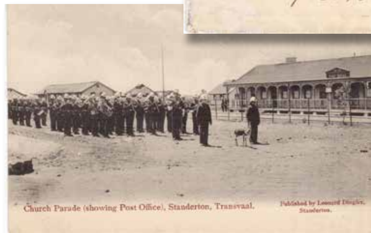
Fig.11: The Standerton Cantonment Post Office.
