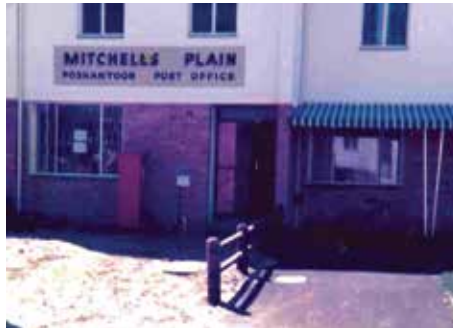
Fig.3: Photograph showing incorrect office name.
